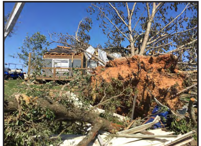
Tornado damage, Onalaska, April 2020. Photo credit: NWS.
